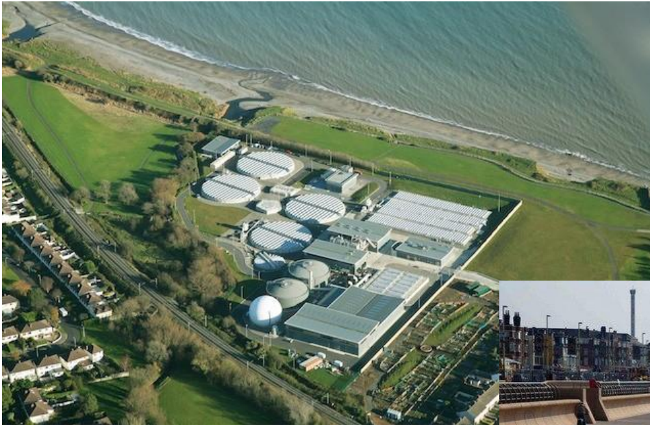
Shanganagh Waste Water Treatment Plant – 50% GGBS
